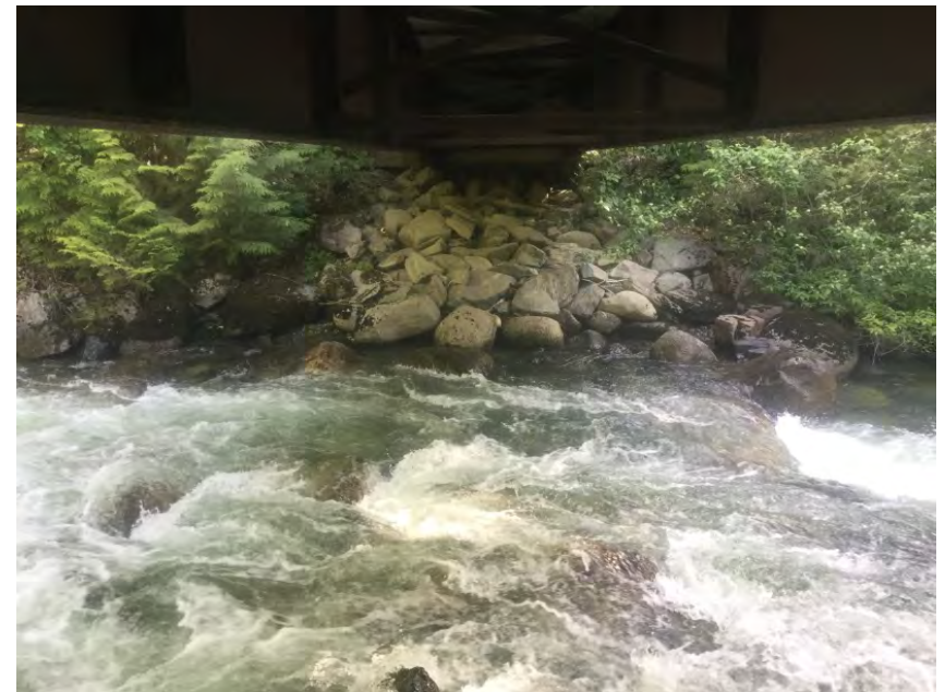
Left Bank Abutment when facing downstream
