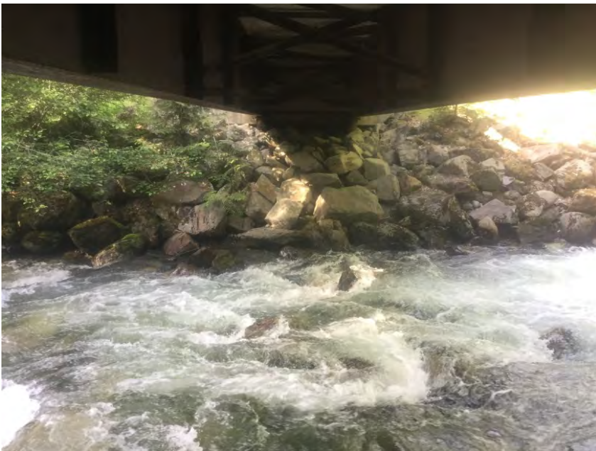
Right Bank Abutment when facing downstream
